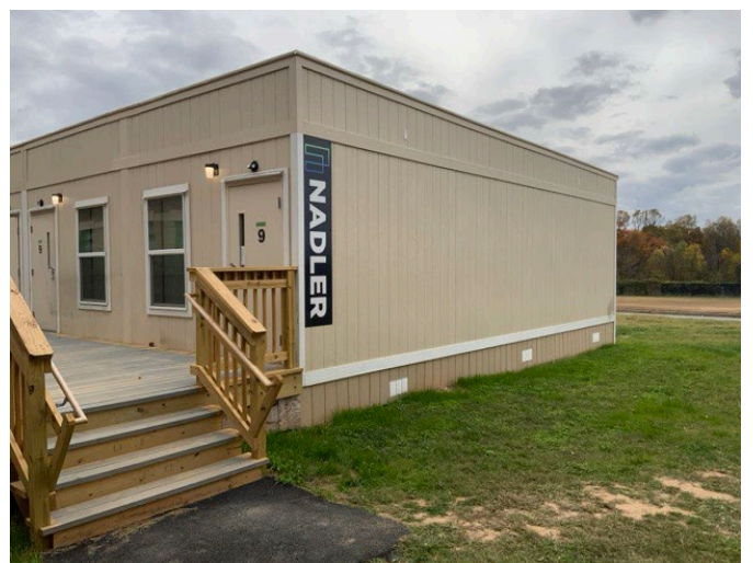
30 - TYPICAL MODULAR BUILDING
