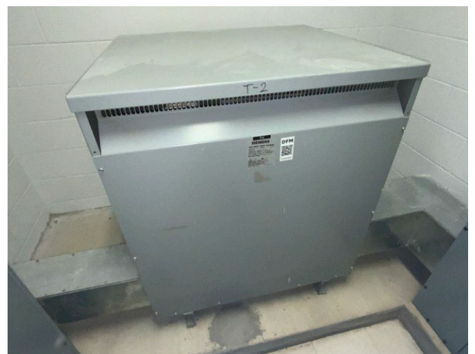
24 - SECONDARY TRANSFORMER
