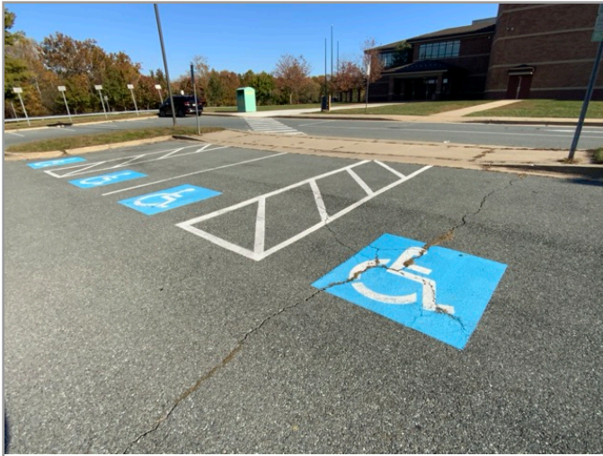
OVERVIEW OF ACCESSIBLE PARKING AREA
