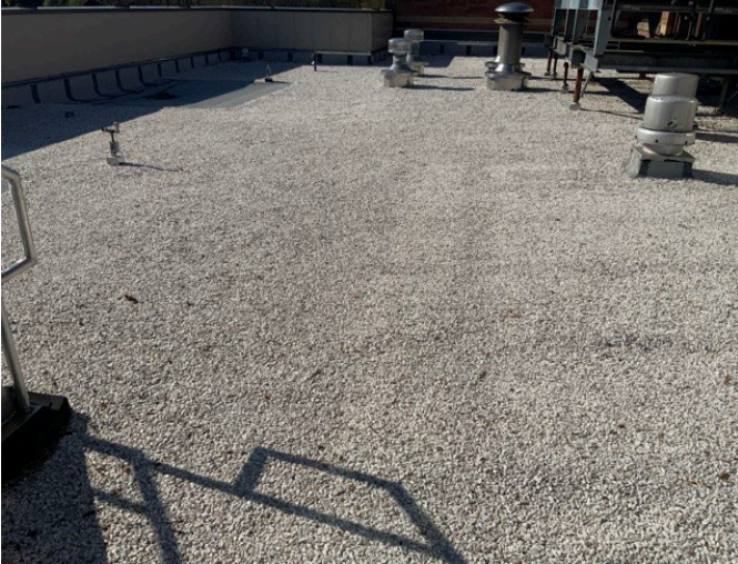
7 - BUILT UP ROOFING
